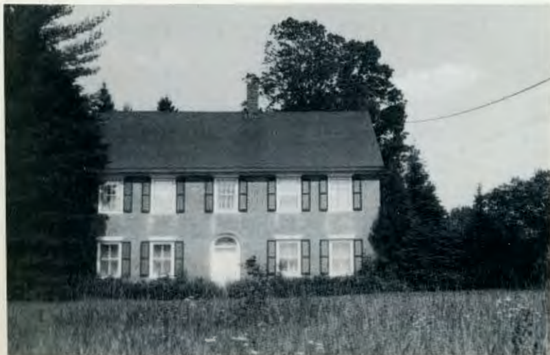
Fig. 9a. Amsden-Hempt House, front (west) . Photograph by the author.
