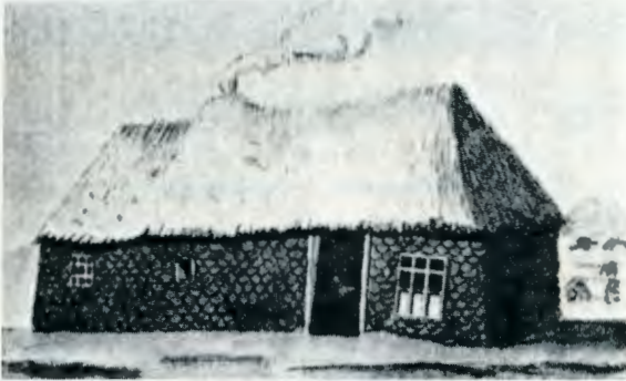
Fig. 6c. Cross passage facade in Scotland. From J. Dunbar, Historic Architecture of Scotland , 1966.
