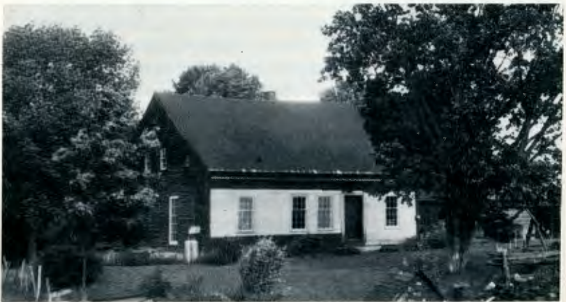
Fig. 6a. Blair House, cross passage facade. Photograph by the author.
