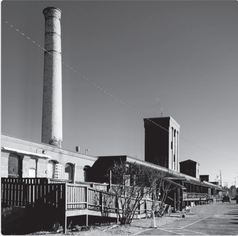
Former Vermont Milk Chocolate Co. factory west side, view looking south, 2024.
