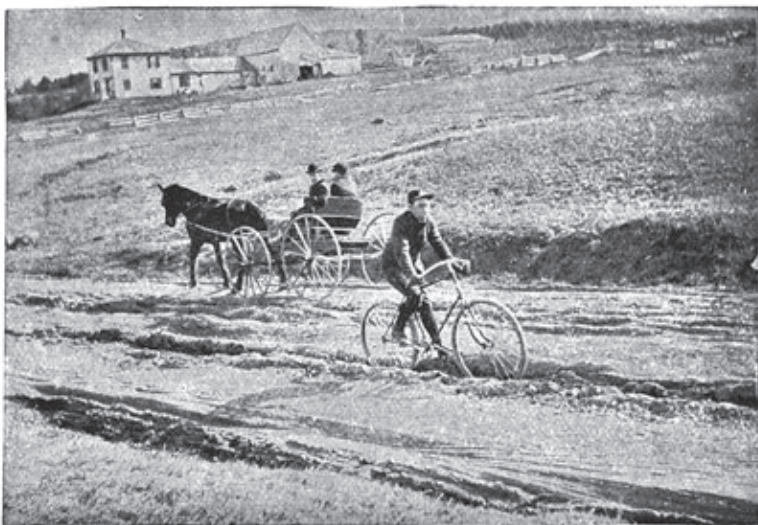
Plate 3.—EFFECT OF NARROW TIRES ON AN UNDRAINED ROAD.
