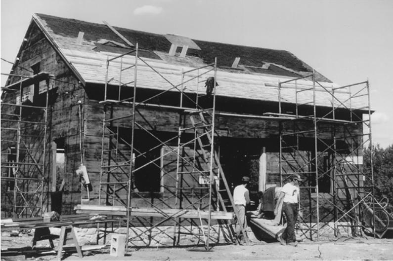
*Ethan Allen Homestead after Ralph Nading Hill's crew removed twentieth-century exterior finishes to reveal original sheathing, and had just begun applying wooden roof shingles. The earliest orientation of the building is indicated by door and window openings. Photograph courtesy of Ethan Allen Homestead Trust.*
