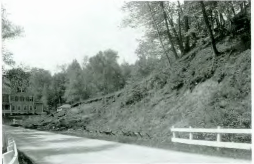
Roadside "raw slopes" (above) where construction and then erosion had taken place, and was likely to continue, were to Taylor "sins" that spoiled "perfect new roads." An old flyer (below) captures his sentiments on the subject perfectly.
